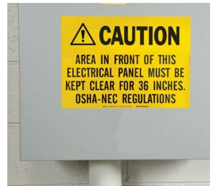
Hazard warning signs
